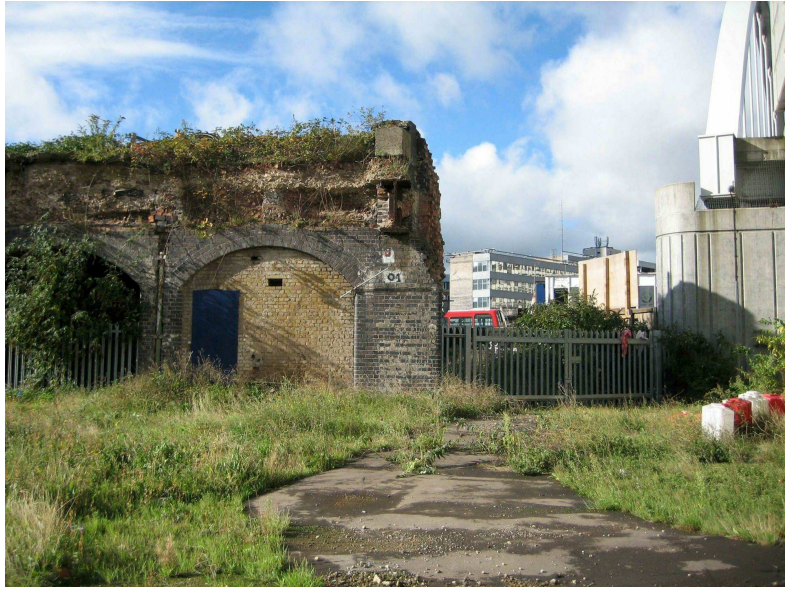
EXISTING NORTH EAST CORNER - Partially collapsed remnants of former arches from previous demolition for the London Overground. Fill material above arches lacks any retaining element to ensure stability of the remaining arches.
